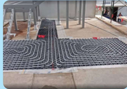
Applications of MRT Cooling System on Mulberry Villa at The Forestias living room floor
