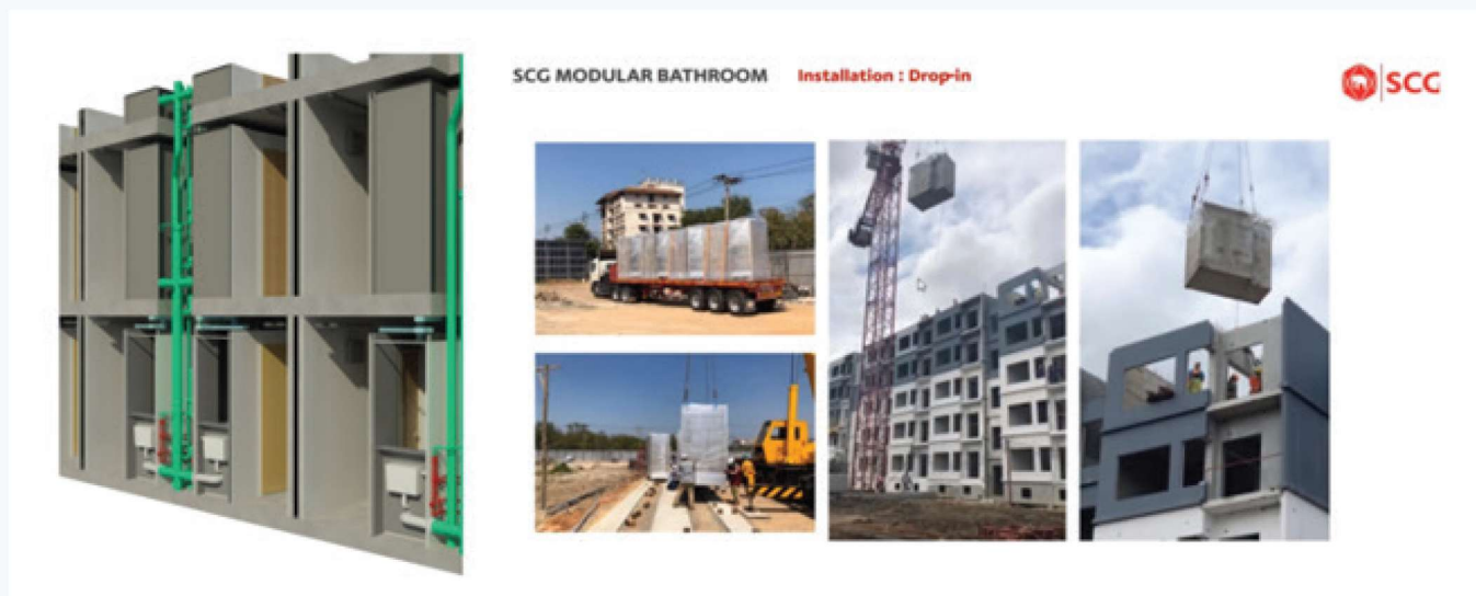
NOVA Patient room Perimeter Modular toilet and Prefabricated sanitary pipe riser
