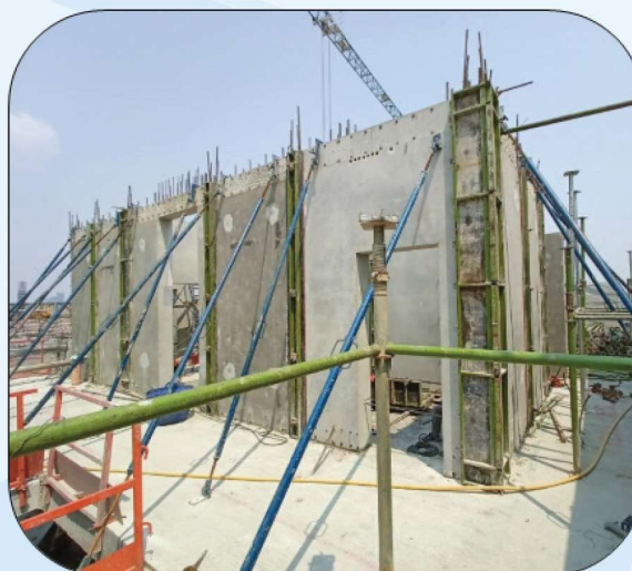
Figure 11 : Construction of HCC Onsite
